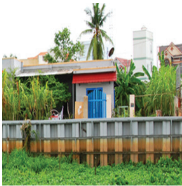
SHEET PILING WITH 2 LEVELS OF ANCHORING
