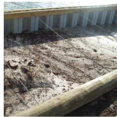
SHEET PILE WALL WITH TIEBACKS
