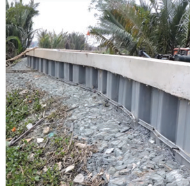
CONCRETE CAP COMPLETION
